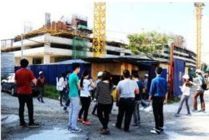
Figure 3: All of us were gathered outside the construction site.
