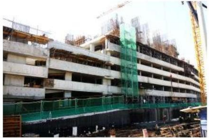
Figure 2: Buildings under construction
