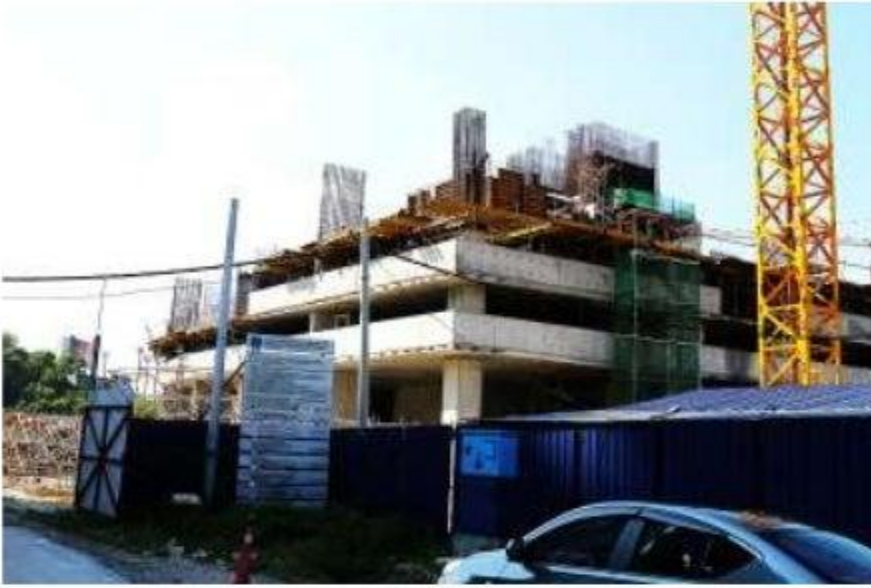
Figure 1: Site Visit to D'Latour Construction Site
