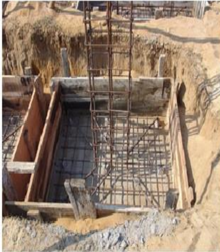
|| || Isolated RCC Footing
